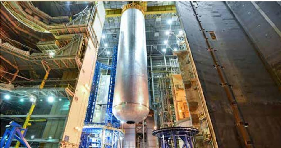
*With welding complete on one more piece of the core stage, the first flight-ready Liquid Hydrogen Fuel Tank for the world's most powerful rocket, NASA's Space Launch System, finishes final welding and is moved off the 170-foot-tall Vertical Assembly Center.*
